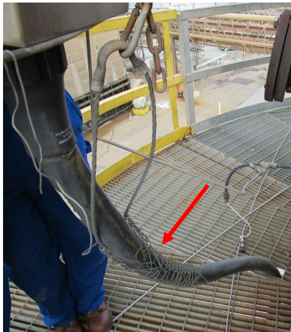
Figure 27 – CEMS traced sample bundle at probe box
