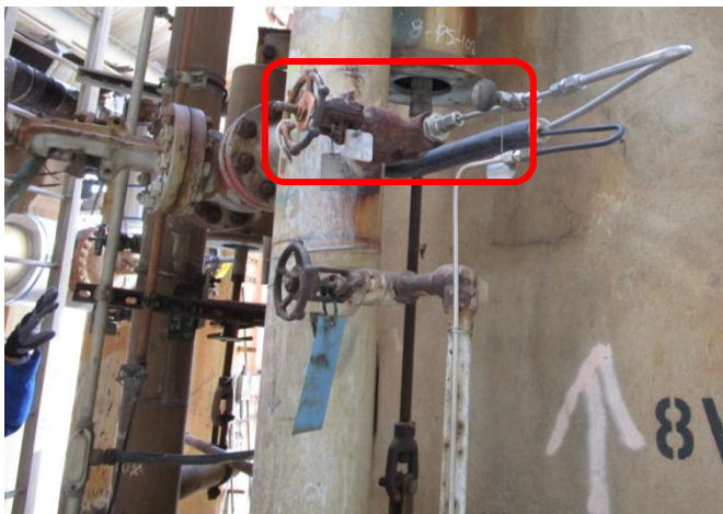
Figure 17 – 868 FCCU Deprop Overhead sample tap
