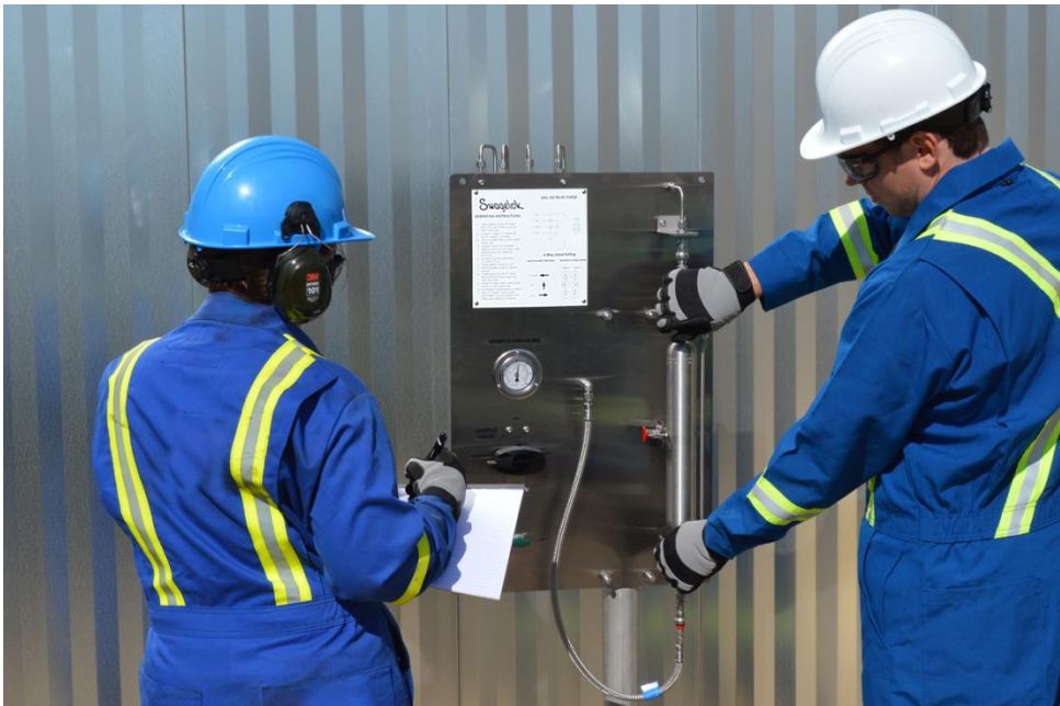
Figure 14 - Safe grab sample station example
