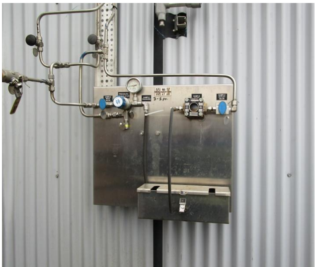
Figure 13 – 137 Crude Unit Foul Gas Sample Station
