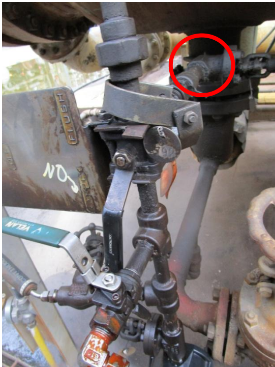
Figure 2 - Sample tap 1: HFO/LFO HXR E-73B
