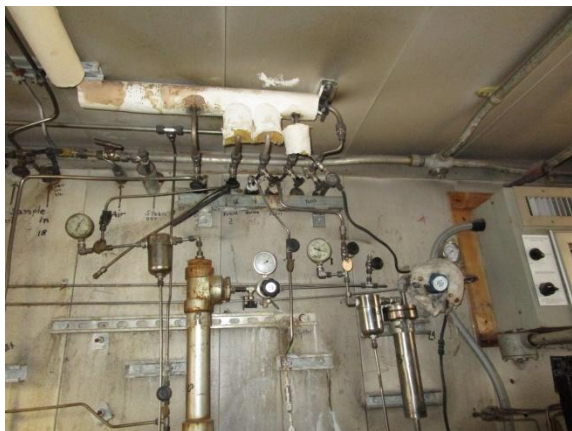
Figure 19 - 868 FCCU Deprop Overhead Sample Conditioning System
